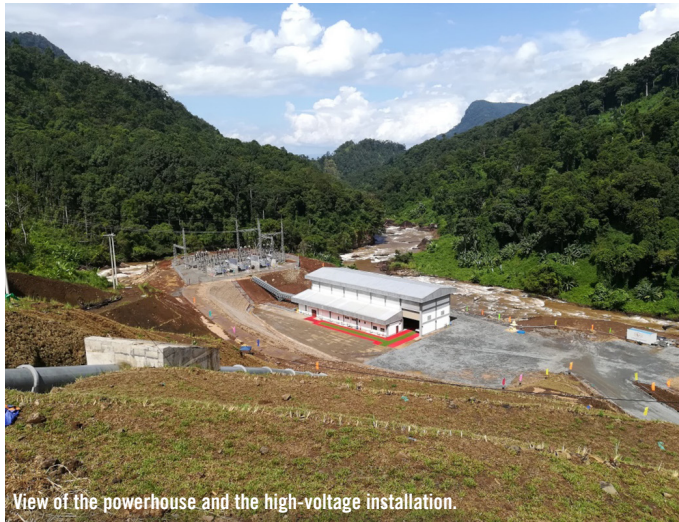
From the transverse structure a 2.7 km long penstock guides the works water down to the turbines in the centre of the plant.
