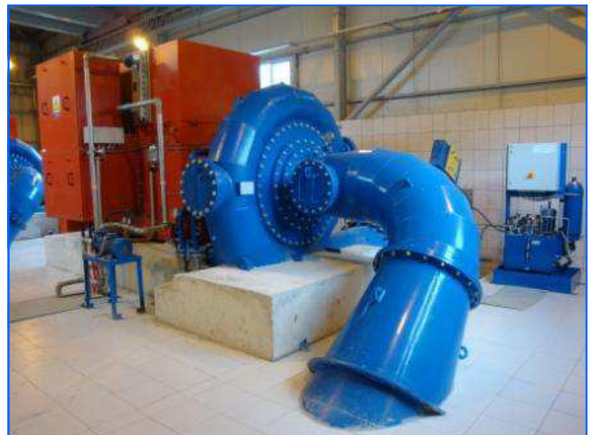
Krafthaus power house
