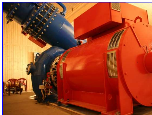
Krafthaus Power house
