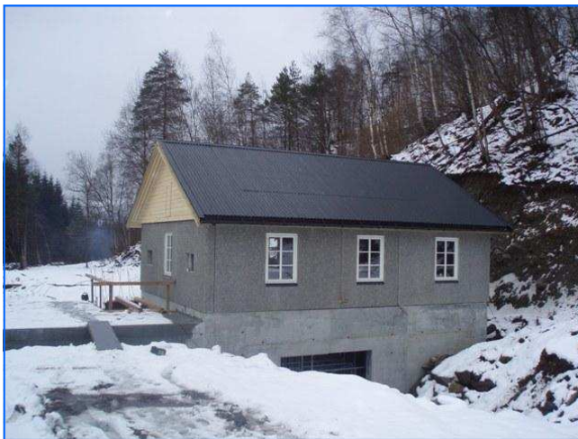
Krafthaus Power house
