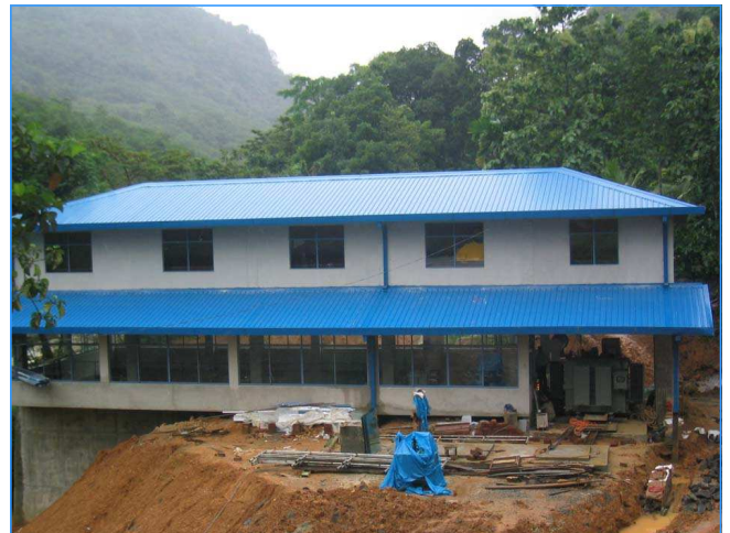
Baustelle in Sri Lanka, Turbinenhaus Construction site in Sri Lanka, turbine house
