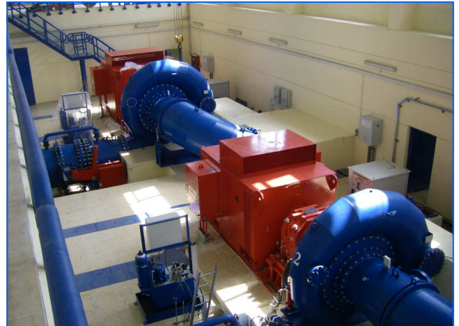
Krafthaus Power house
