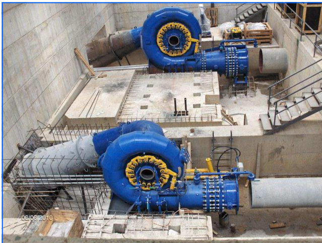
Baustellenmontage turbine installation
