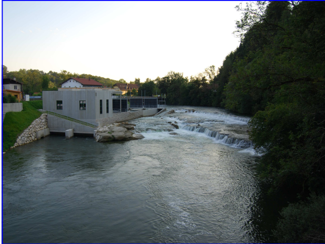
Krafthaus Power house
