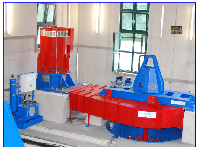
Kaplan Turbine Kaplan turbine
