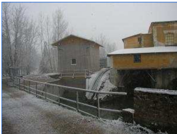
Turbinenhaus Power House
