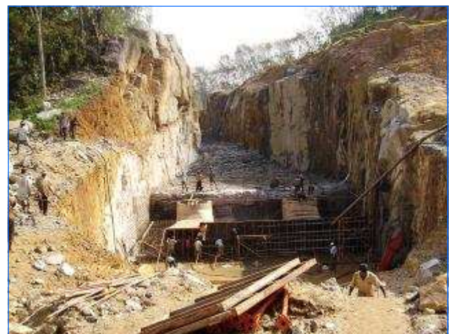
Baustelle Jänner 2007 Construction site in January 2007
