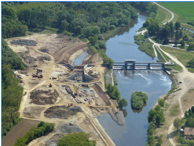
Baustelle Mai 2007 Construction site in May 2007
