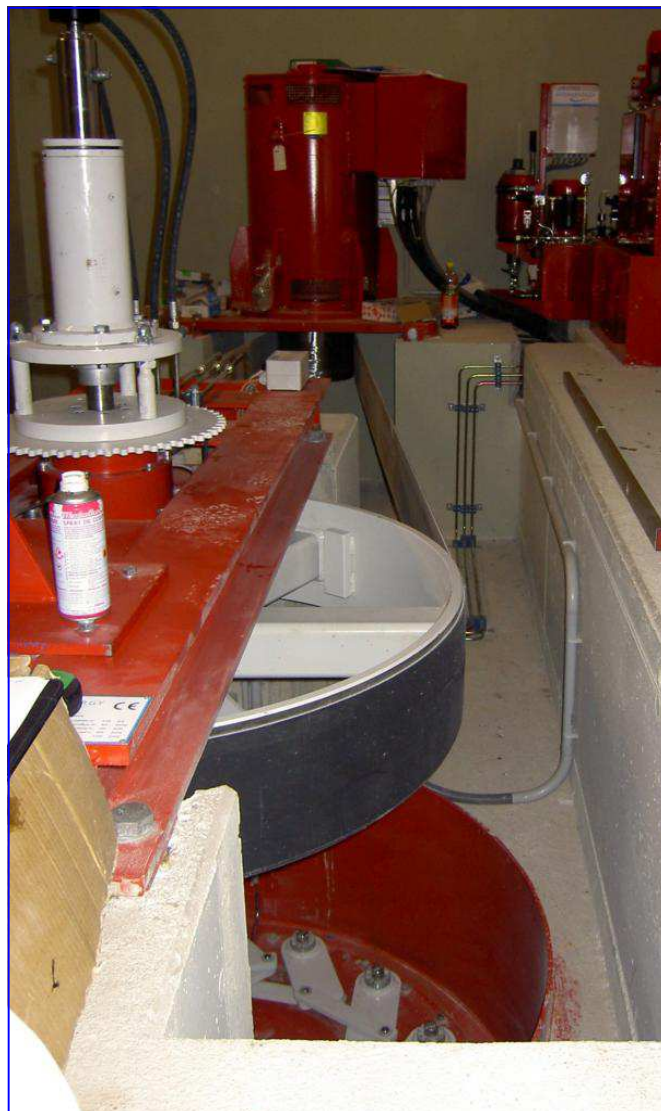
Krafthaus Power house
