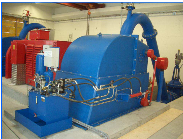
Krafthaus Power house
