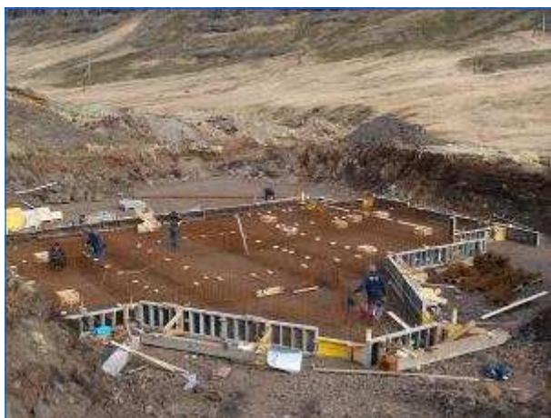
Baustelle Turbinenhaus Construction site power house
