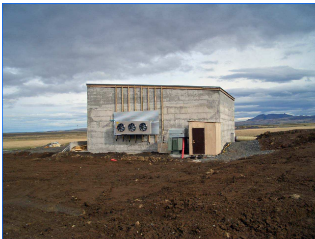
Turbinenhaus in Island Turbine house on Island
