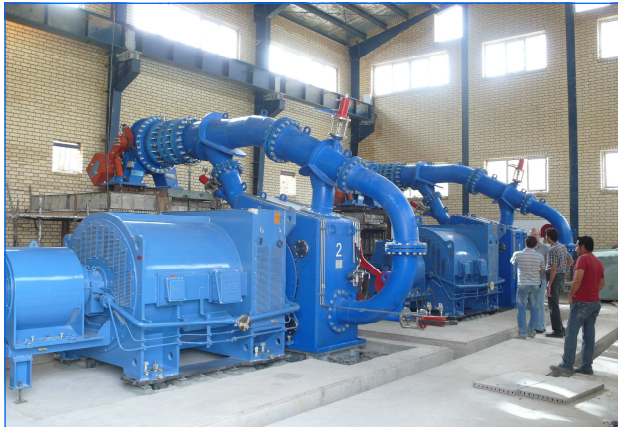
Installation der Pelton-Turbinen Installation of Pelton turbines
