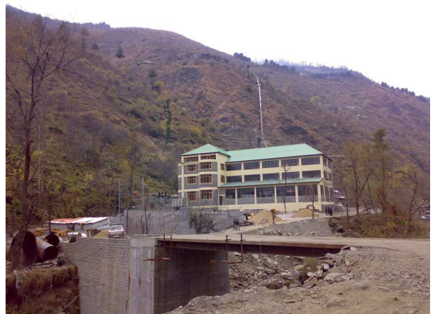
Turbinenhaus in Indien Turbine house in India
